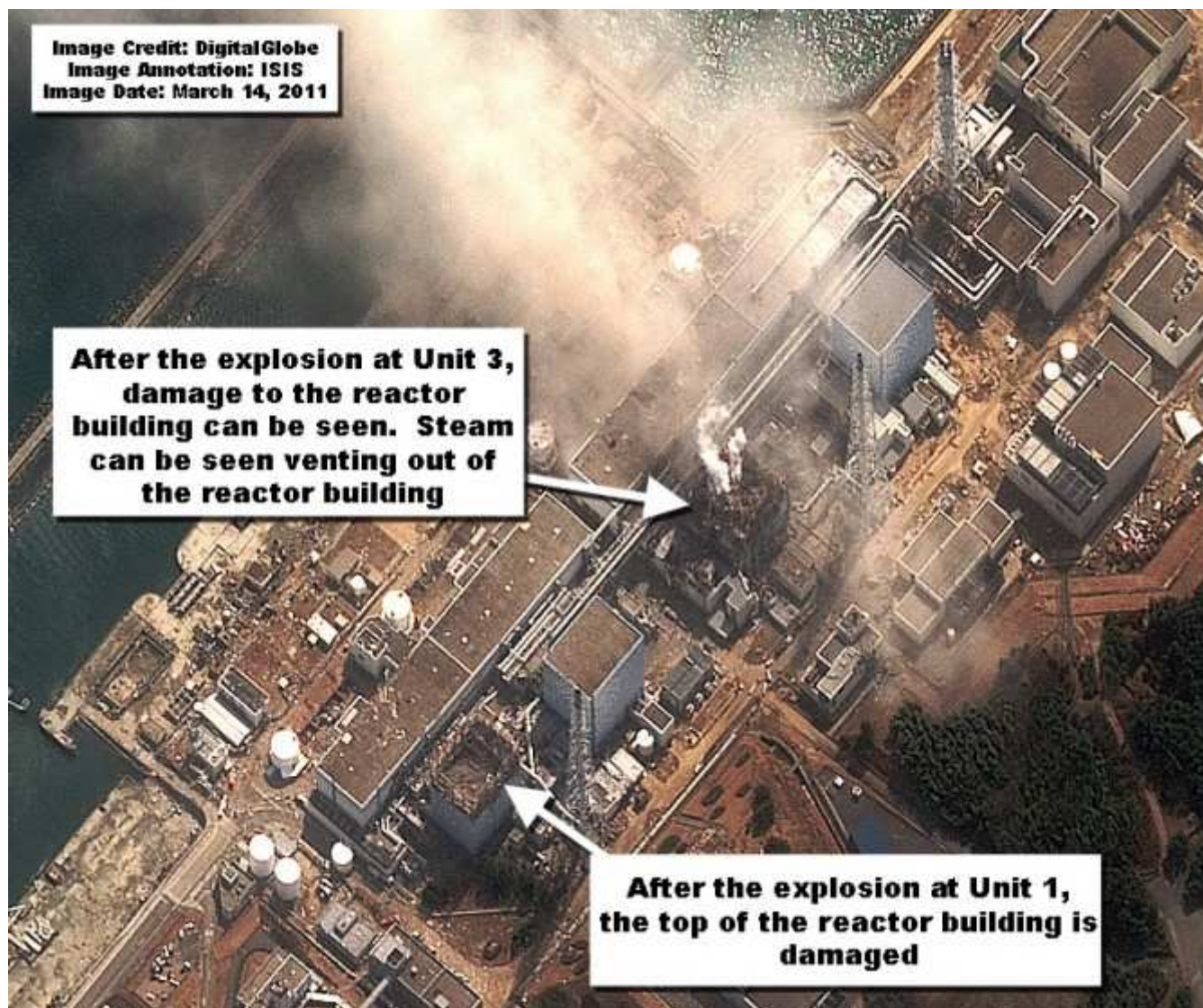
Figure 1. DigitalGlobe image from March 14, 2011 of the Fukushima Daiichi reactor site. Damage to the reactor buildings for Units 1 and 3 can be seen in this image. Steam can be seen venting out of the reactor building for Unit 3.
